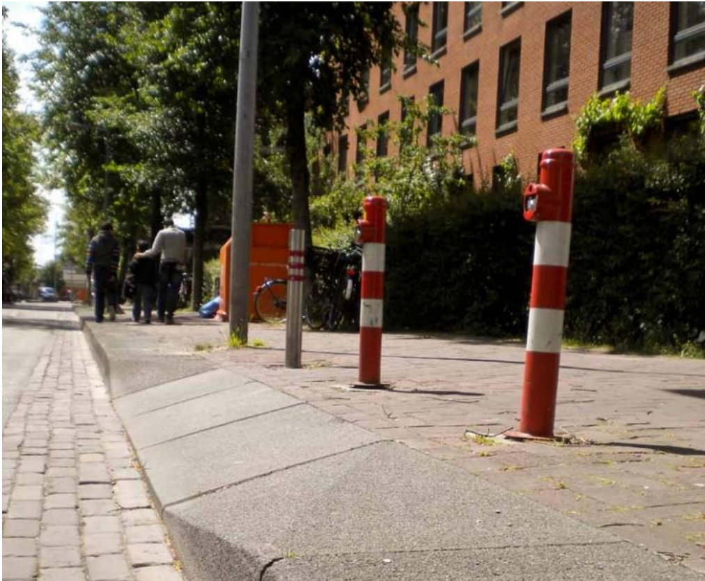
Figure 4-19: Bollards and raised curbs prevent motor vehicles from entering GWL Terrein
