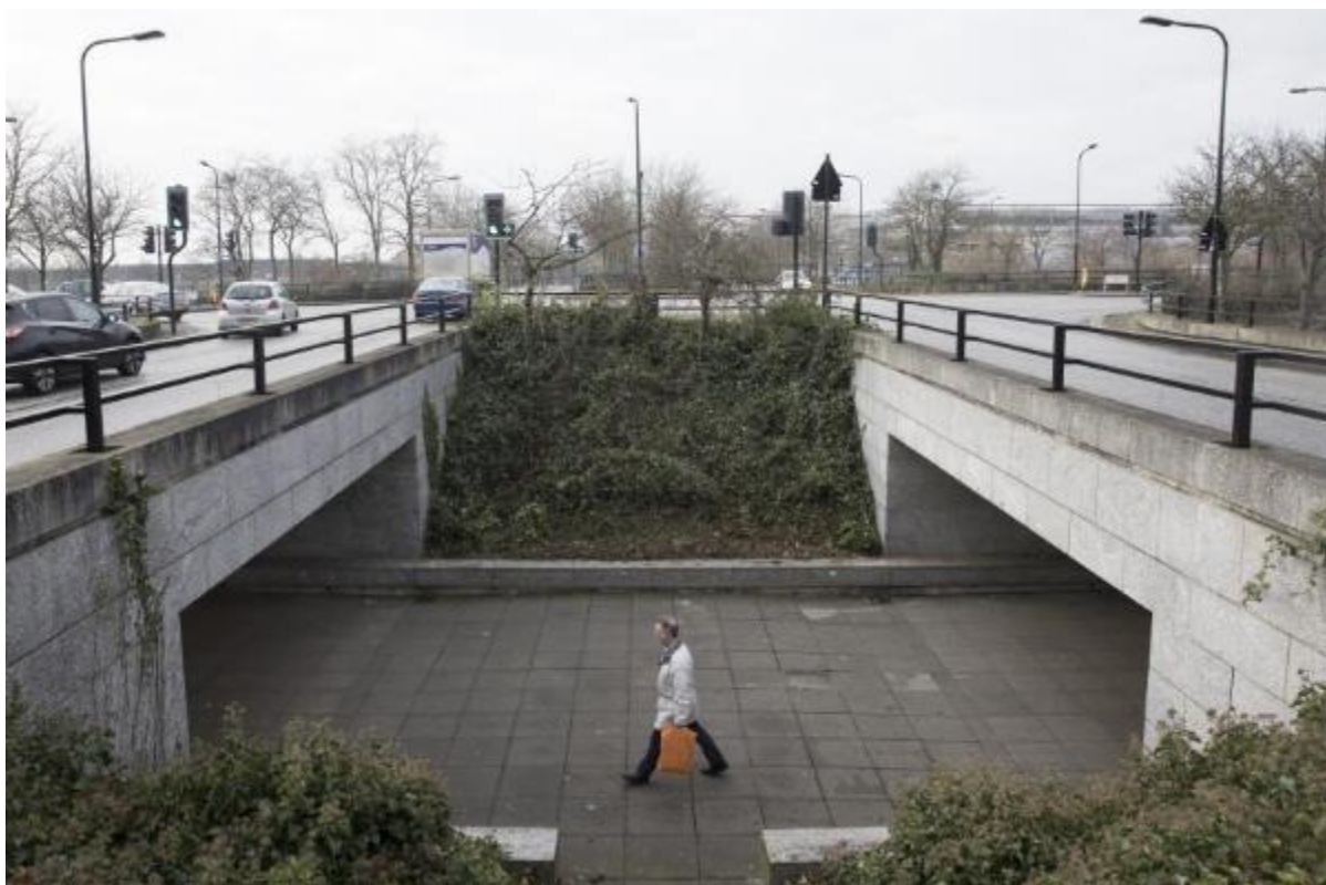
Figure 5-1: An underpass in Milton Keynes
