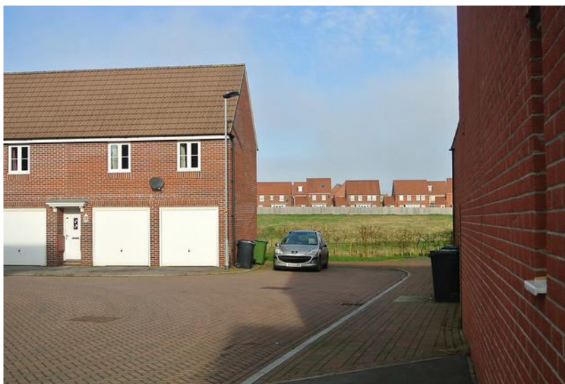
Figure 4-1: An example of public realm dominated by car access considerations (Clackers Brook, Melksham)
