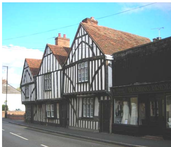
Fig. 85 Nos 23-27A Bridge Street.
