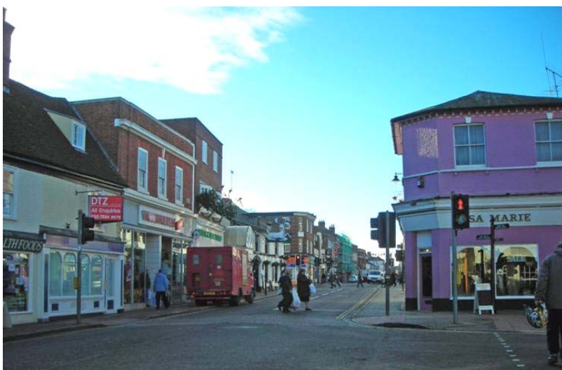
Fig. 13 Newland Street looking south-west with no. 40, Lisa Marie, projecting forward on the line of encroachment on the medieval market place.
