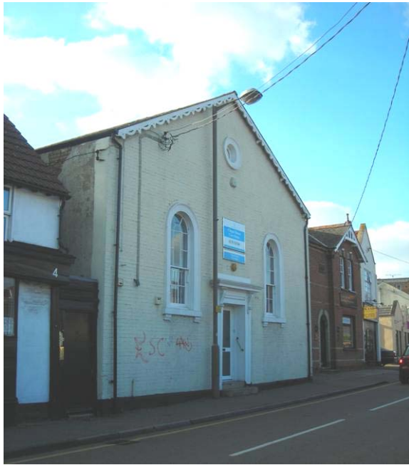
Fig. 94 Former Baptist chapel, Maldon Road.
