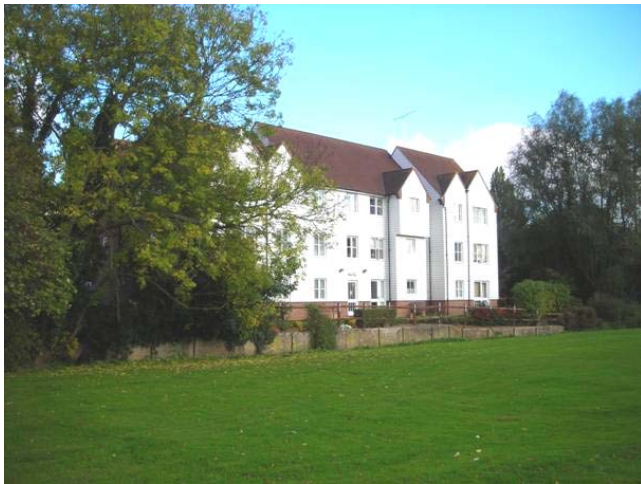
Fig. 80 Moorfield Court viewed from the bridge.
