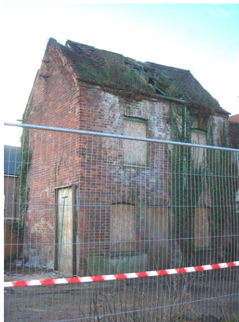
Fig.100 Brick building surviving behind no. 137 Newland Street.
