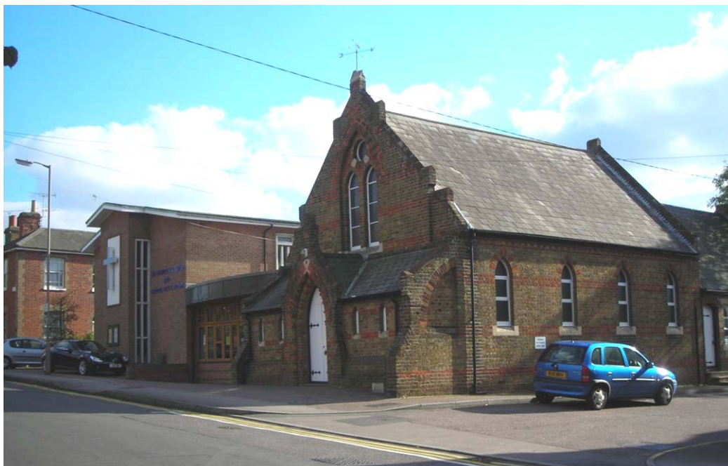
Fig. 88 Methodist church and church hall, Guithavon Street.
