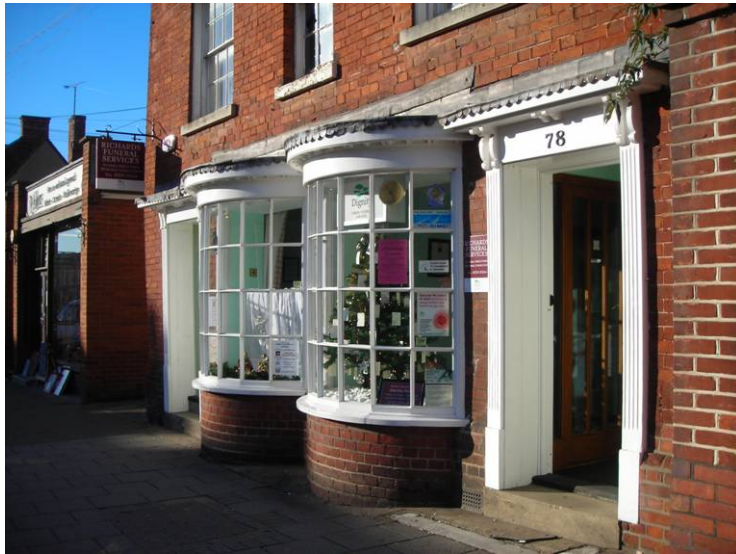
Fig. 33 Georgian-style bow shop front with small panes and ornamental cornice.
