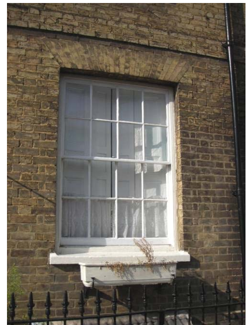
Fig. 29 Gauged brick window head, sliding sash window with fine glazing bars. This window also has timber internal folding shutters.
