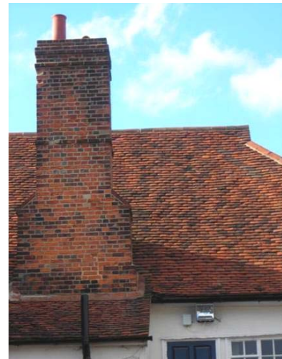
Fig. 30 Clay peg tile roof.
