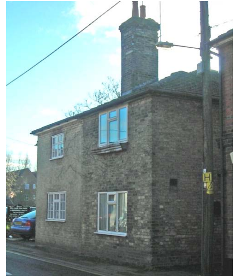
Fig. 101 Cottage in Mill Lane with unsympathetic replacement windows.
