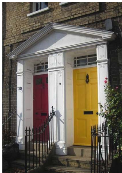
Figs 31 & 32 Panelled door with ornate iron fanlight and fine gauged brick arch (left), and pedimented doorcase with simple rectangular fanlights (right).
