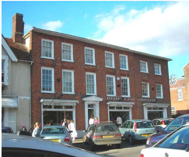
Fig. 57 Nos. 90-92 Newland Street, Byfords.
