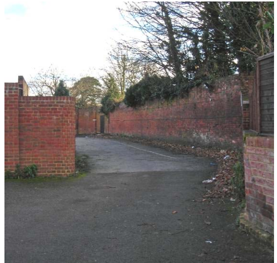
Fig. 34 Brick boundary walls in Spread Eagle yard.
