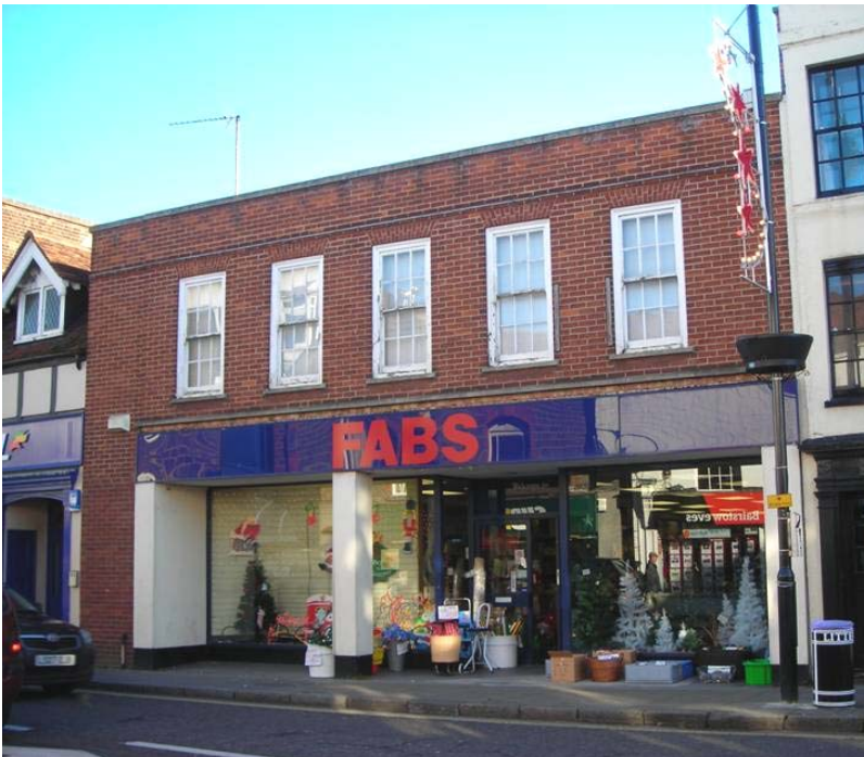
Fig. 96 Shiny, reflective materials are unsympathetic in conservation areas.
