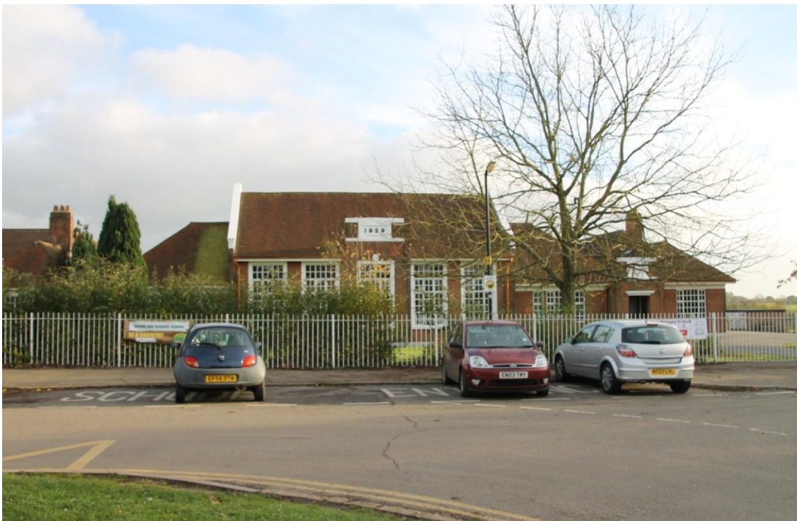
Fig. 7 View of Silver End School
