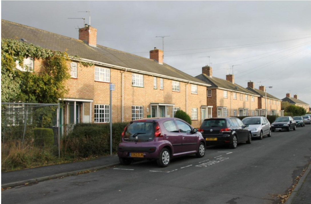
Fig. 12 View of the terraced housing on Grooms Lane
