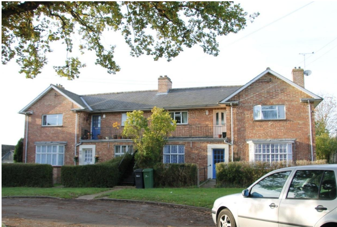
Fig. 8 View of a block of flats on Leicester Court
