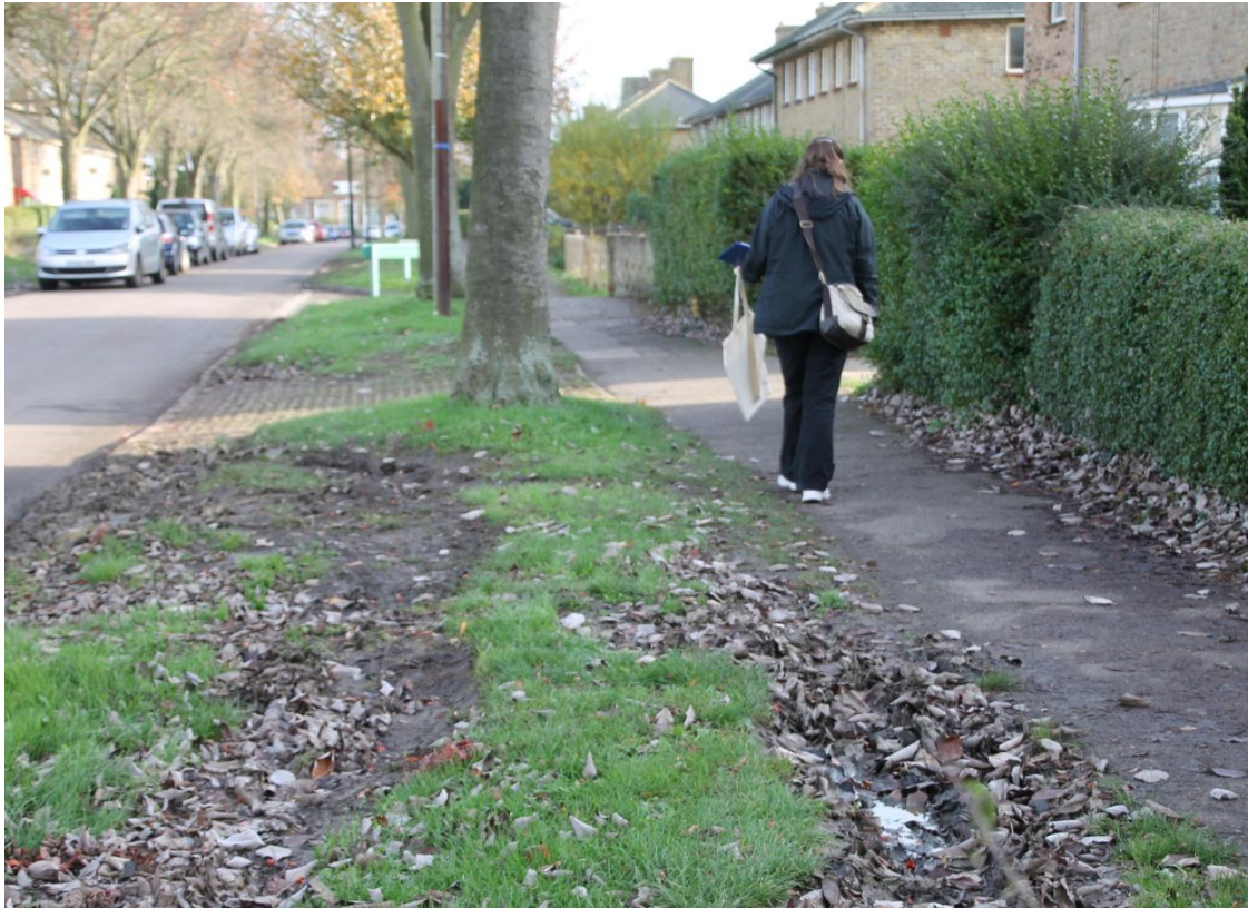
Fig. 9 View of verge damage in Valentine Way
