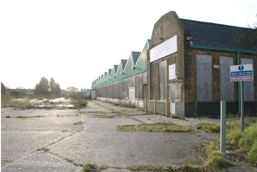
Fig. 14 The former Crittall Works factory, looking along the line of the saw-tooth roof
