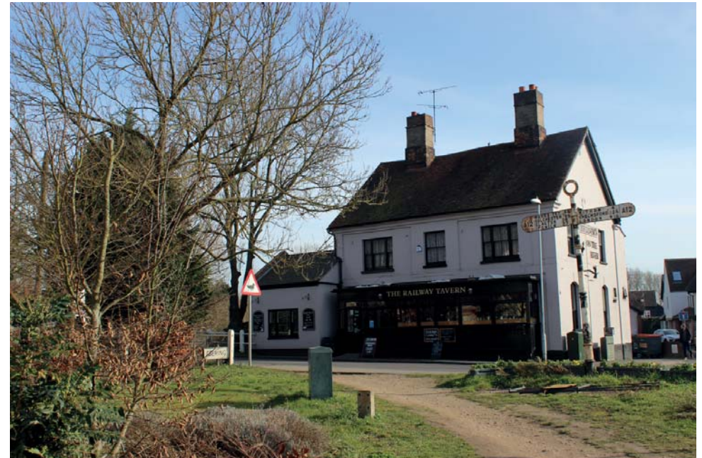
Figure 34 View of The Railway Tavern and historic signpost
