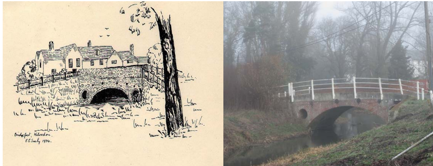
Figure 26 View north of road bridge (ERO Imp 141-1-2) also showing Mill in its setting
