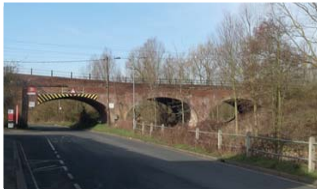
Figure 29 View northwards to railway viaduct across the blackwater
