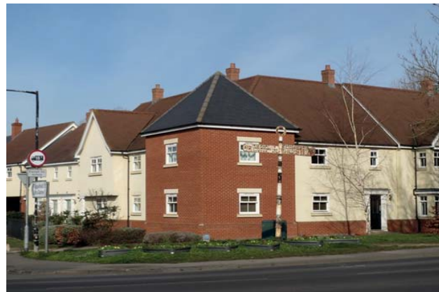
Figure 15 View of 'neutral' modern development at road junction
