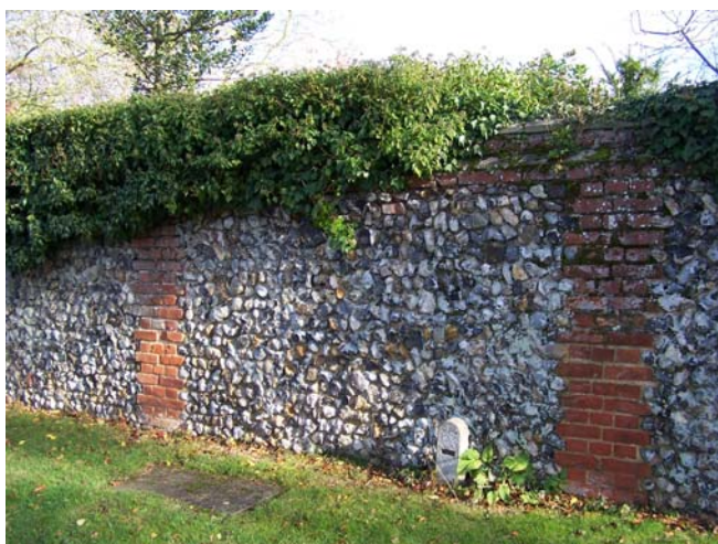
Figure 5 Wall to the Old Vicarage.
