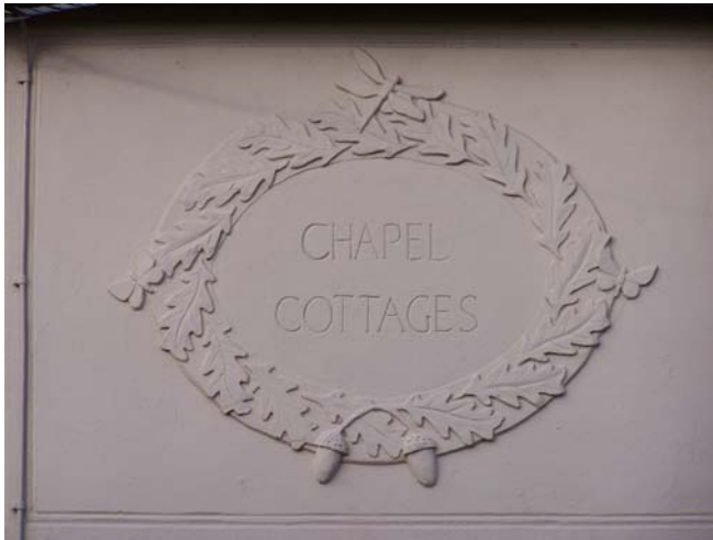
Figure 27 Parget detail on Chapel Cottages.
