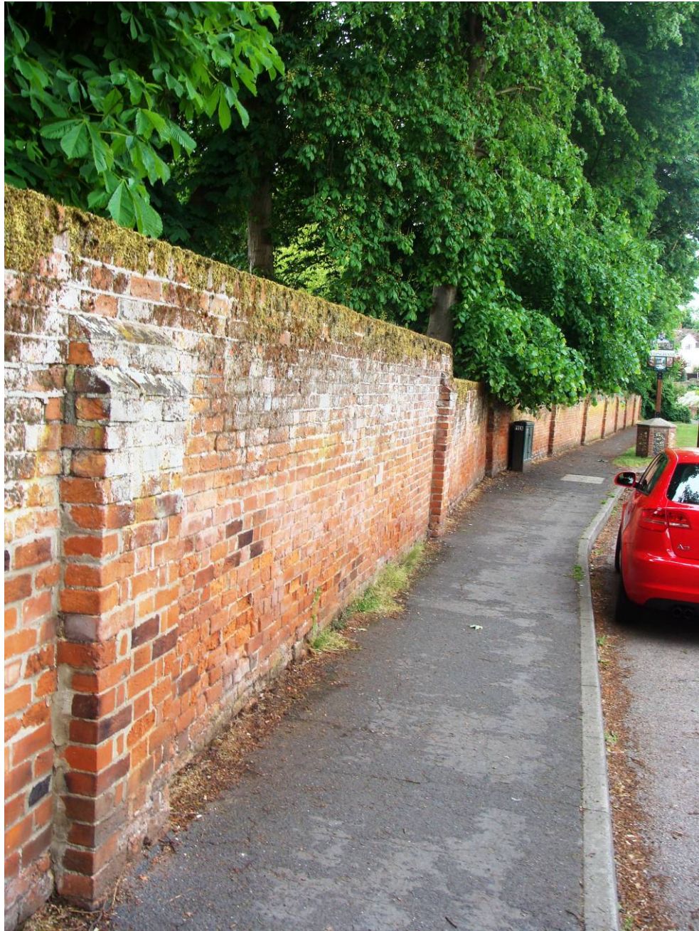
Picture 20 Old Rectory boundary wall
