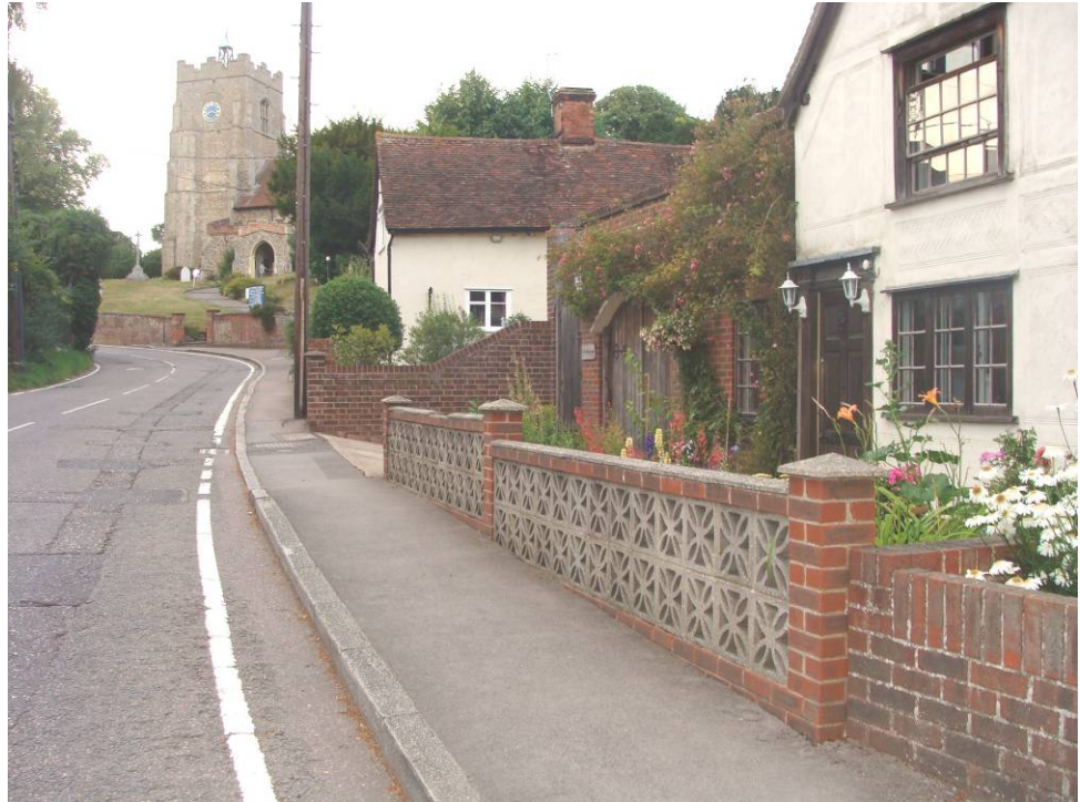
Picture 23 Inappropriate boundary detail
