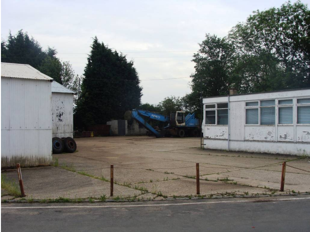
Picture 14 Dilapidated buildings at industrial site
