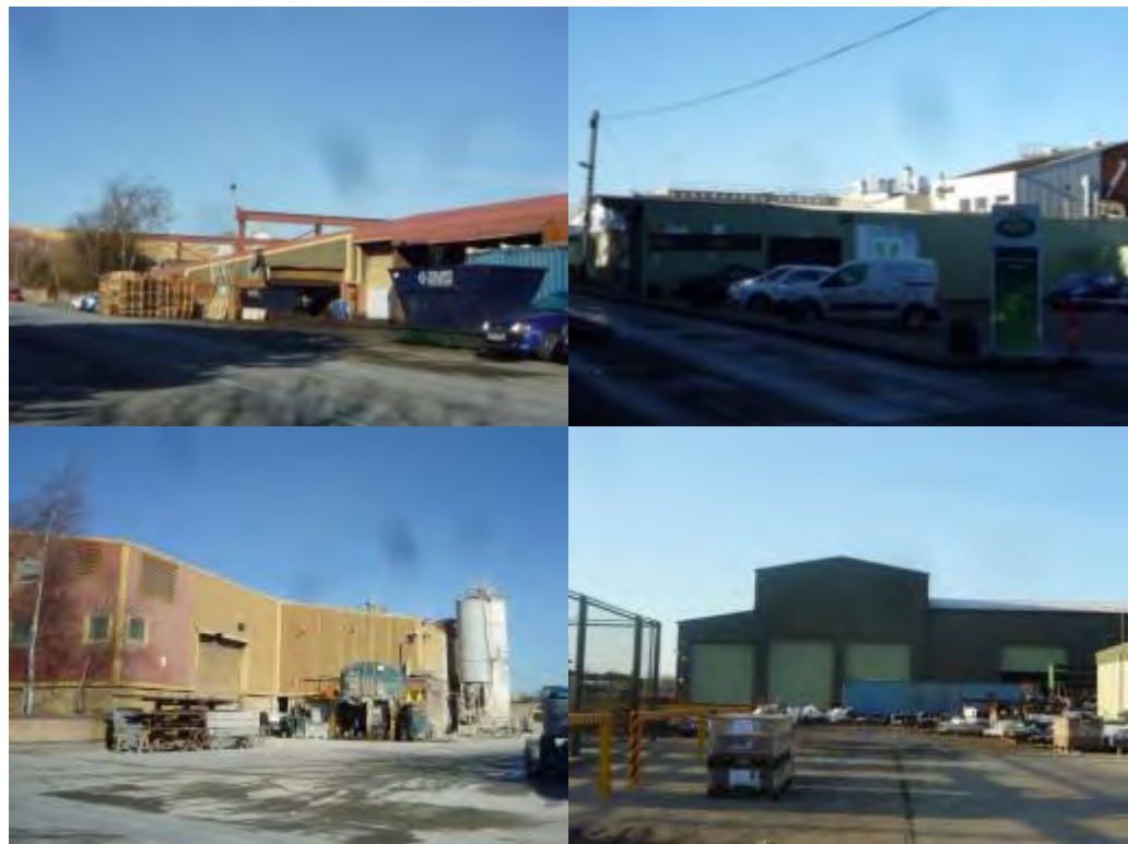
Source: AECOM (2015). Locations from top left clockwise: Earls Colne Airfield (C14); Arla Factory, Hatfield Peverel (C25); Gosfield Airfield (C8); Earls Colne Airfield (C14).
