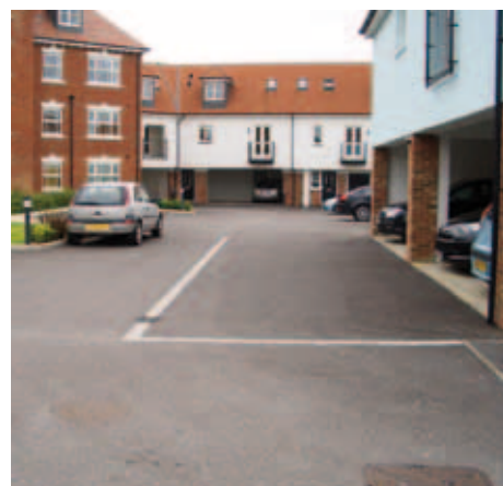
Visible undercroft parking
