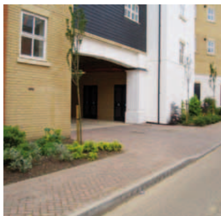
Undercroft secure parking (gated entry).
