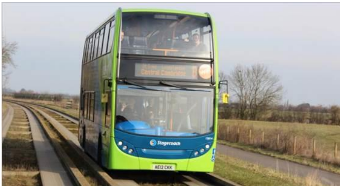
Figure 4-10: Cambridgeshire Guided Busway (Source: Prismall, 2016)
