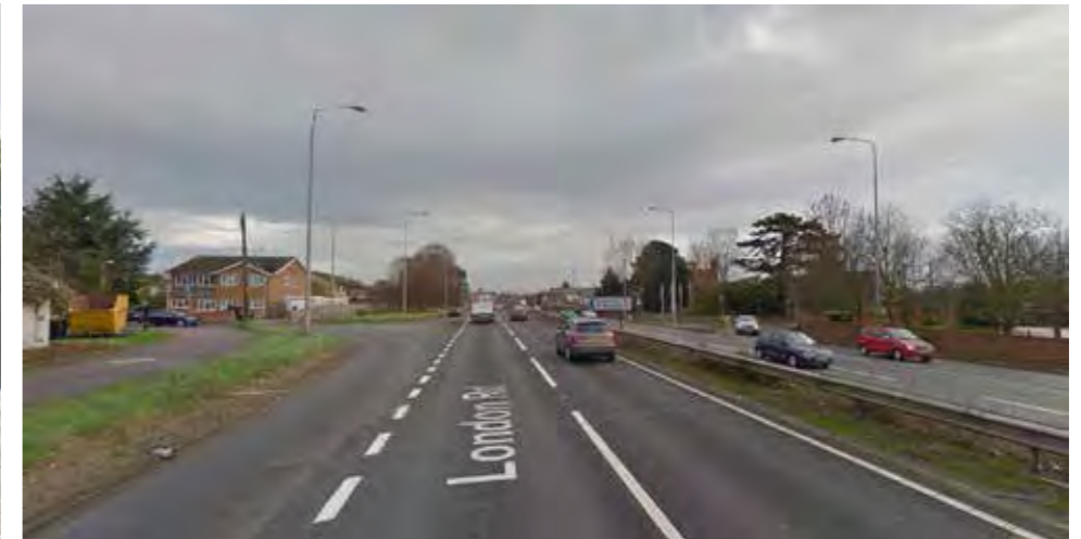
Figure 18: Street view of the A12 North of Witham
