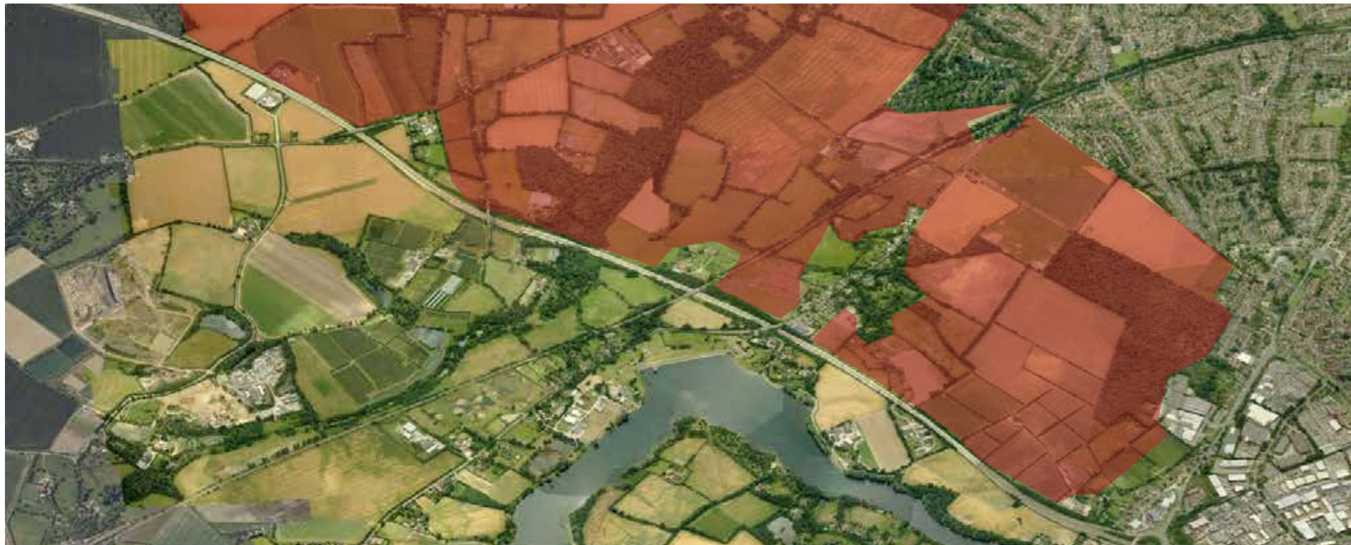
Figure 41: View across north section of the Site Area looking south with Ardleigh Reservoir in the foreground and Severalls Industrial Park in the bottom right corner. Source: Bing Maps Bird's Eye View
