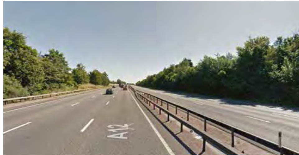
Figure 19: Street view of the A12 North of Chelmsford
