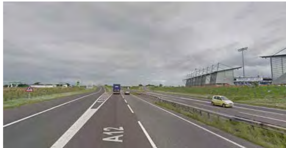
Figure 16: Street view of the A12 approach to junction 28
