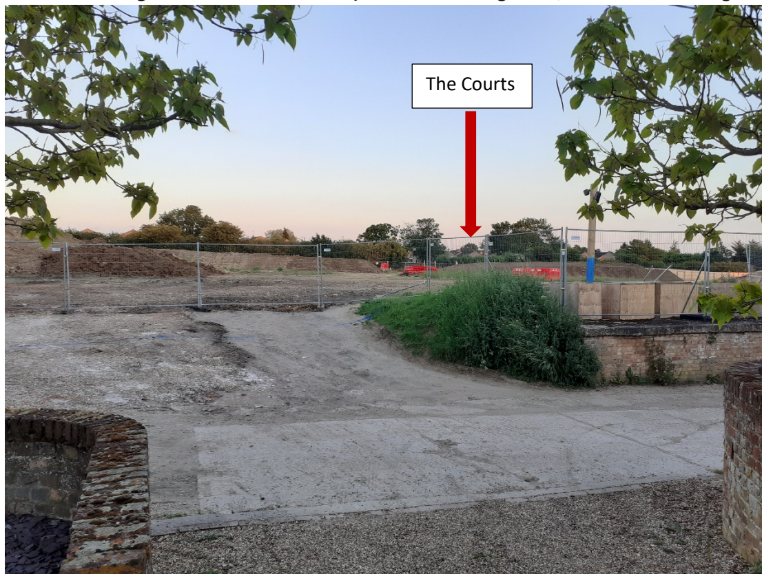
c. View looking S towards Conrad Road (WITN426 in mid ground, The Courts in background)
