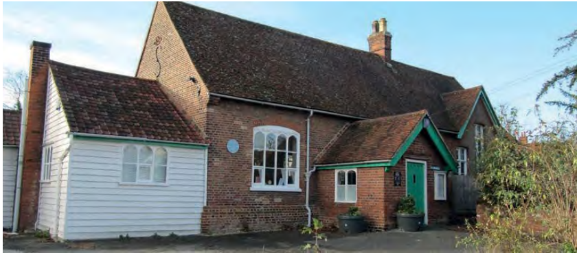
Former Ayletts Foundation School , currently the library and museum
