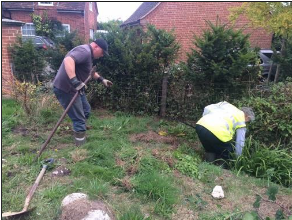
Clearing ditches within the Parish
