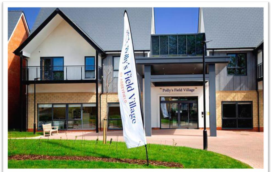
45 affordable units were provided at Polly's Field Retirement Village in Bocking by Abbeyfields
