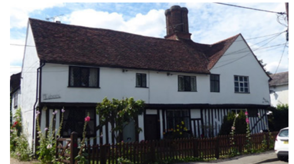
Figure 62 Exposed framing at 35 and 37 Church Lane, dating to the early sixteenth century
