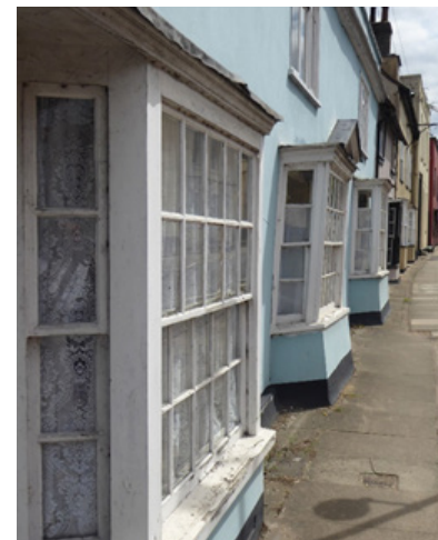
Figure 63 Bay window shopfronts added to a refaced sixteenth to seventeenth century building, 54-56 Bradford Street.
