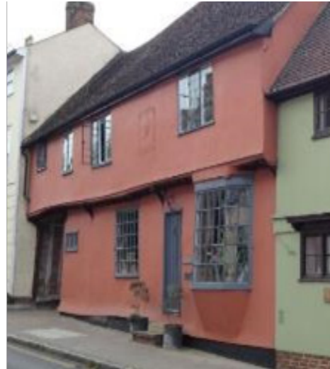
Figure 39 The jettied Dragon House, 41 Bradford Street
