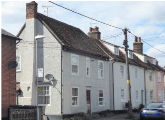
Figure 57 The former Spread Eagle Public House
