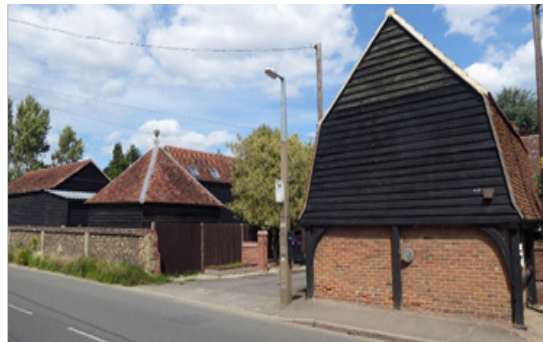
Figure 60 Agricultural buildings of the former Boleyn's farmstead
