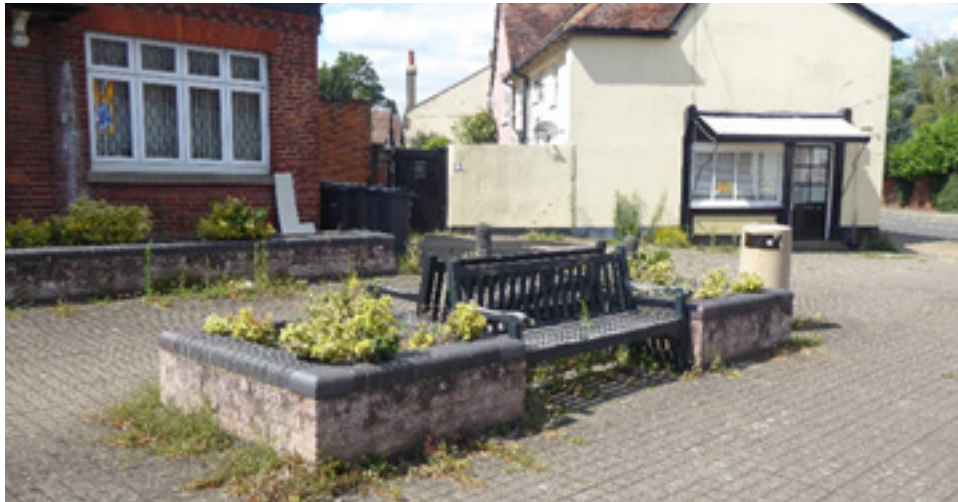
Figure 82 The small public piazza in front of the former Six Bells Public House
