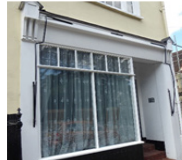
Figure 61 A nineteenth century shopfront at 15 Bradford Street
