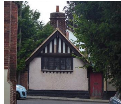
Figure 51 37A Bradford Street
