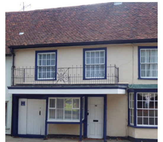
Figure 64 An eighteenth-century bay shop window on posts with a canopy in seventeenth century building at 92 Bradford Street
