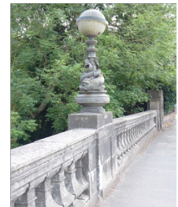
Figure 25 A lamp on the Bridge over the River Blackwater
