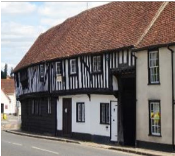
Figure 40 Close studding 114-118 Bradford Street
