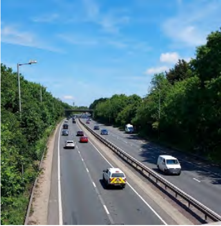
A12 looking towards Witham
