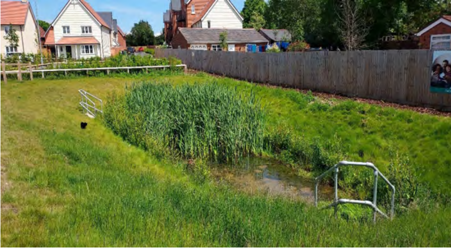
SuDS area at Mulberry Green
