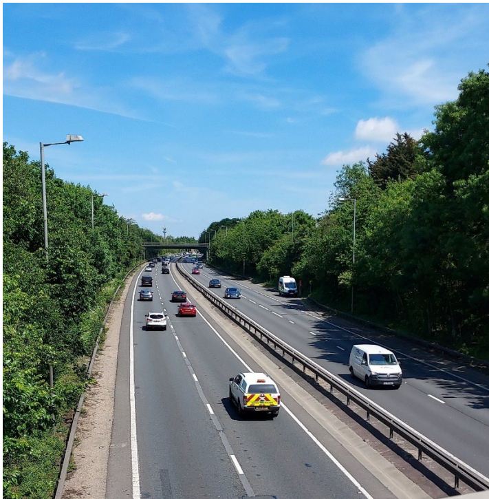
A12 looking towards Witham
