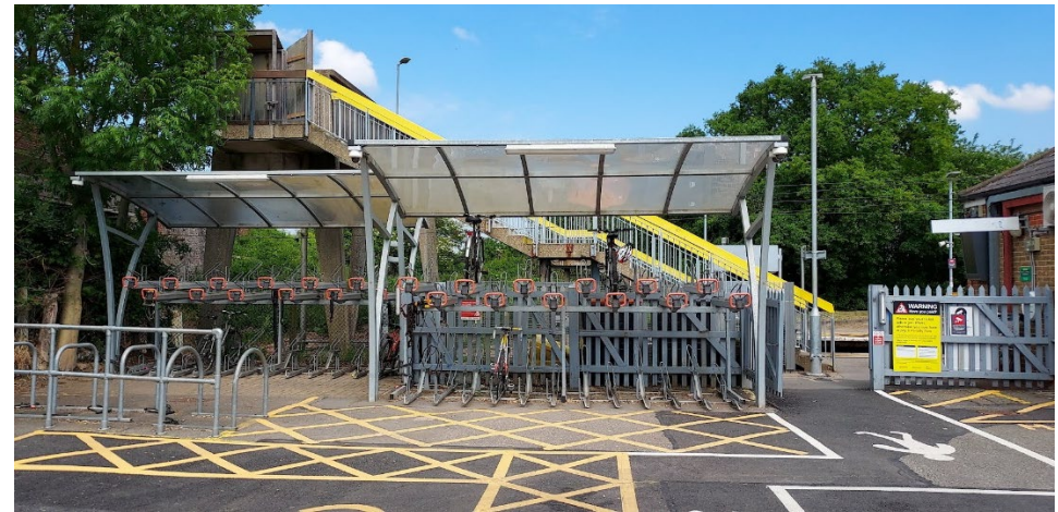
Cycle Storage at Station
