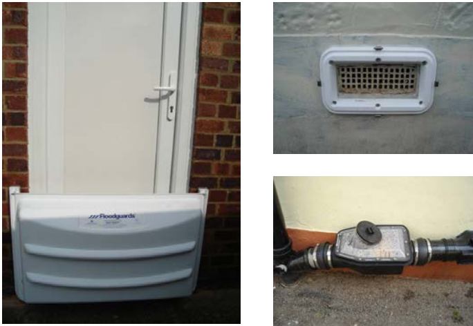
Figure 6-3 Examples of flood barriers, air bricks and non-return valves
