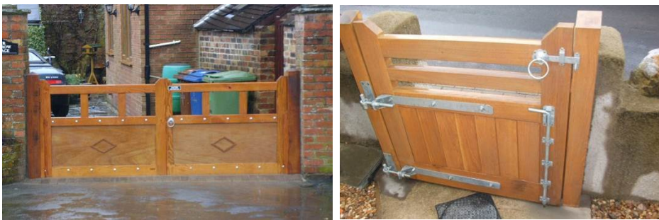
Figure 6-4 Example of flood gates
